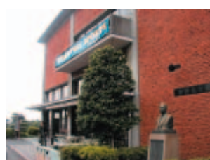
Construction of combined wing (Fujiyama Memorial Hall)
