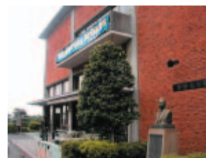
Construction of combined wing (Fujiyama Memorial Hall)
