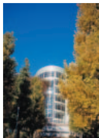
Sousoukan Building on Yagami Campus
